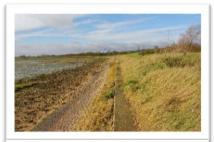
against future coastal erosion. Where possible, previously removed and preserved materials, including the Armorloc blocks, were re-used in order to reduce wastage and maintain the client's budget. The refurbishment works resulted in a significantly improved appearance to the embankment, as well as a durable coastal defence structure.
